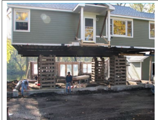
Figure 2.21 2008 Elevation of home on Fox River in Sheridan
