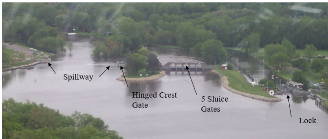
Figure 2.13 Stratton Dam, before improvements
