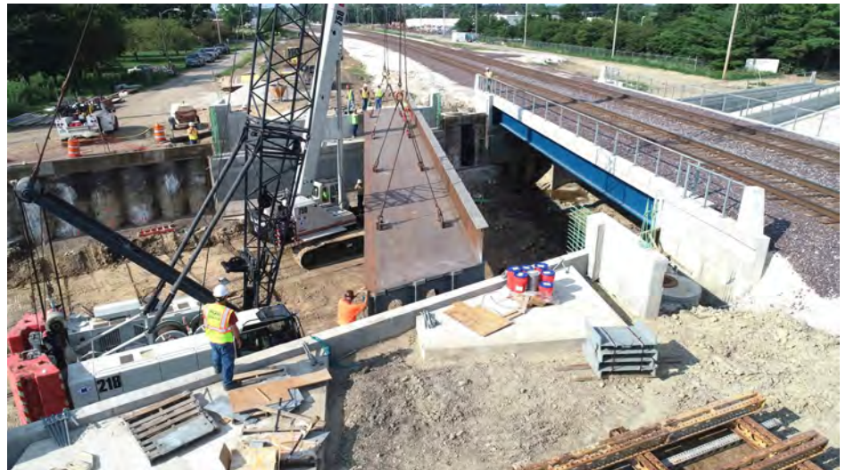
Work on the Springfield rail relocation project. PHOTO Hanson Professional Services
