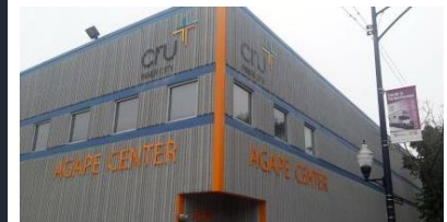
Agape Community Center
